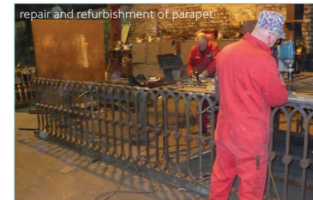
repair and refurbishment of parapet
