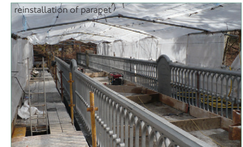
reinstallation of parapet
